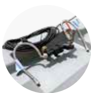
Roof Mounted Auto Water Switch Controller, Mains Water Isolation Valve + SS Connection Hoses
